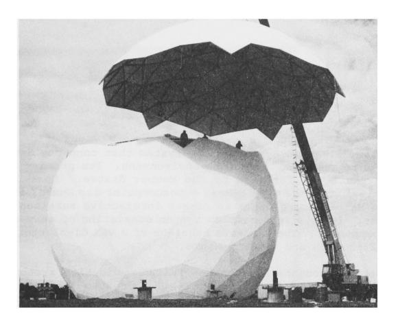
Fig. 4: Radome of a ground station in its final stages of construction
